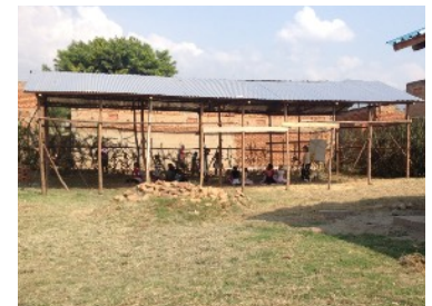
Sunday School Structure
