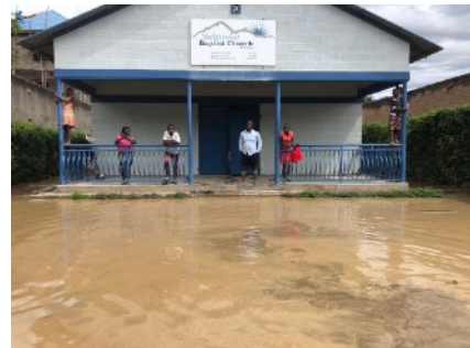
Flooding around the church
